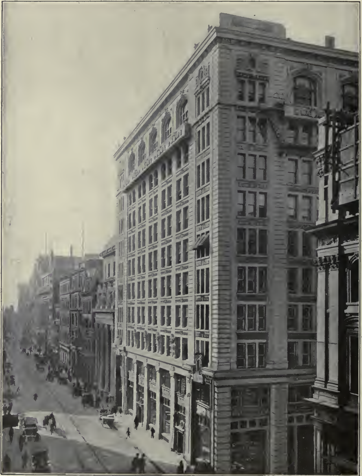
North side of St. James Street to-day. The heart of the financial district, showing the Dominion Express Building, the Royal Bank of Canada, the Canadian Bank of Commerce and several other prominent buildings.
